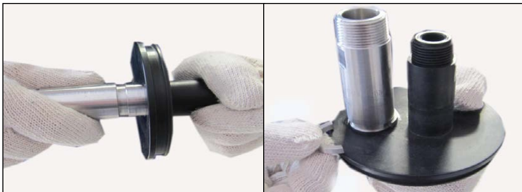
Figure 2.13 Feed/concentrate port installation.
