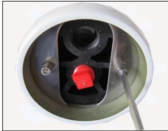
Figure 2.13 Install locking kit segment
