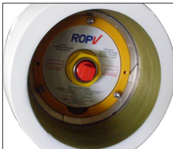
Figure 2.24 Install permeate port plug
